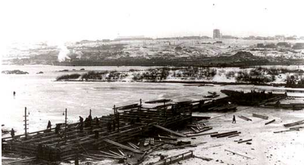
Fig. 2. Construction of the intersection between the Dnieper's banks
