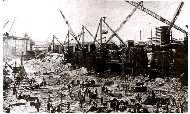
Fig. 3. Construction of formwork for concrete laying
