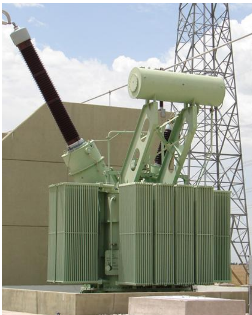
Figure 1.1 - Single-phase shunt reactor POM 50000/500
